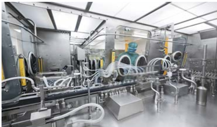
The Halle expansion includes the installation of a new commercial filling line with two freeze dryers as well as a clinical filling line with an additional freeze dryer. Both the new commercial and clinical lines are equipped with automated loading/unloading, capping and inspection infrastructure, designed to support international manufacturing and regulatory requirements.
